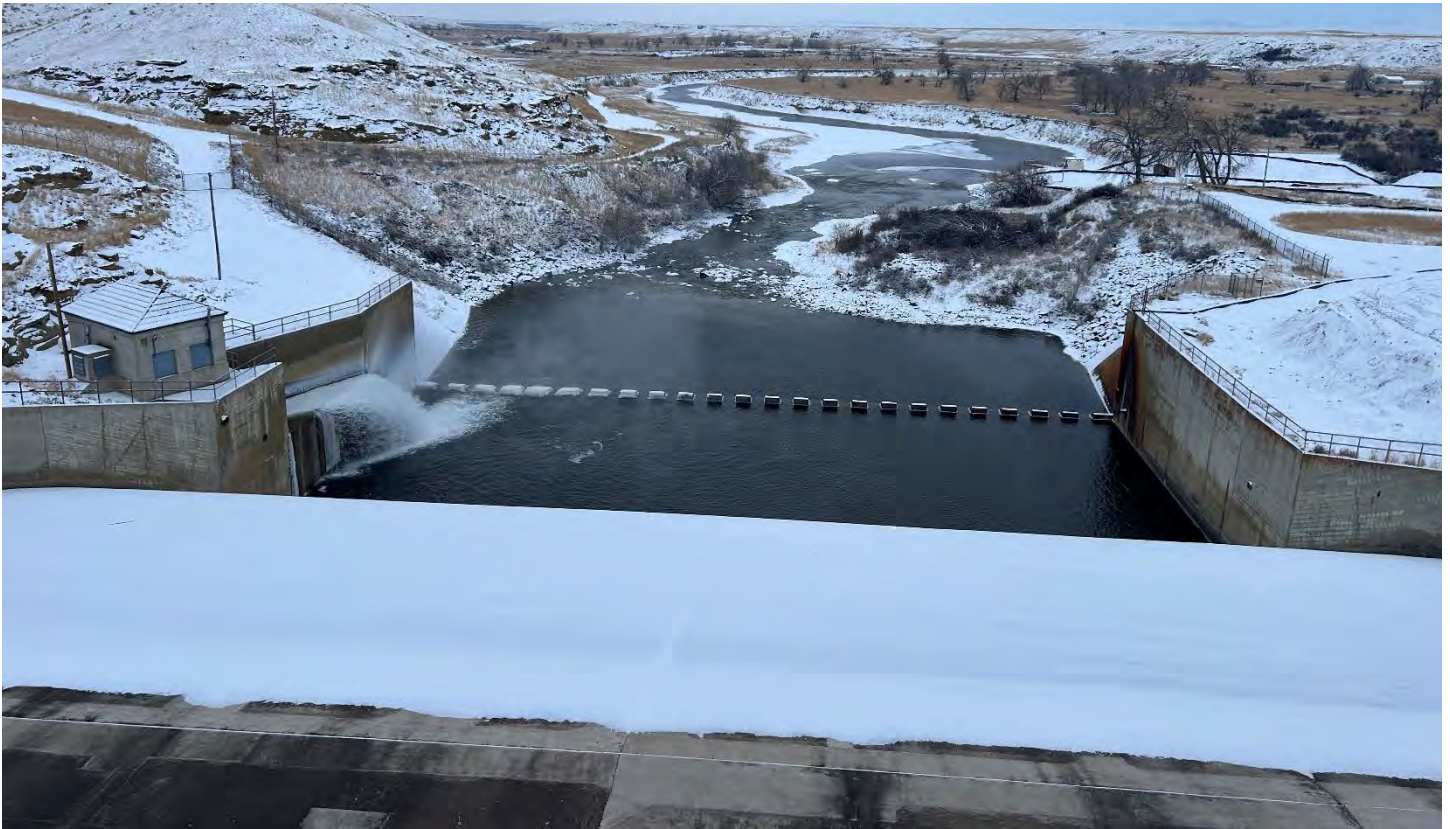
Downstream of Fresno Reservoir, January 2025
