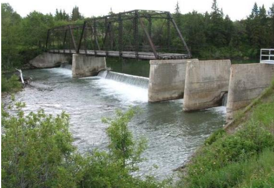
Figure 2-1. St. Mary Diversion Structure 1
