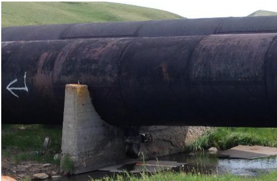
Figure 2-6. Halls Coulee Saddle Support
