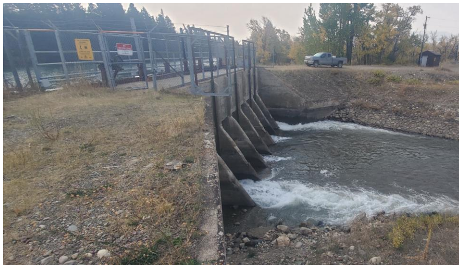
Figure 2-2. St. Mary Diversion Structure Headgates
