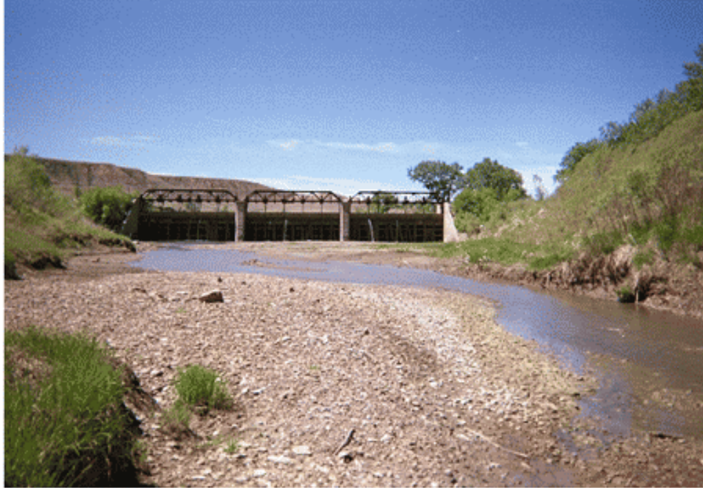
Photo 3.2 - Vandalia Dam, operated by the Glasgo Irrigation District.
