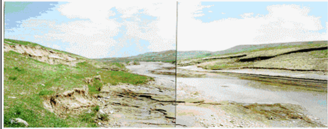
Photo 4.1 - Landslides along the St. Mary Canal.
