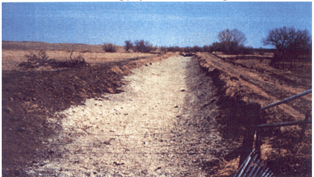
Photo 5.1 - Canal lining project in the Zurich Irrigation District.
