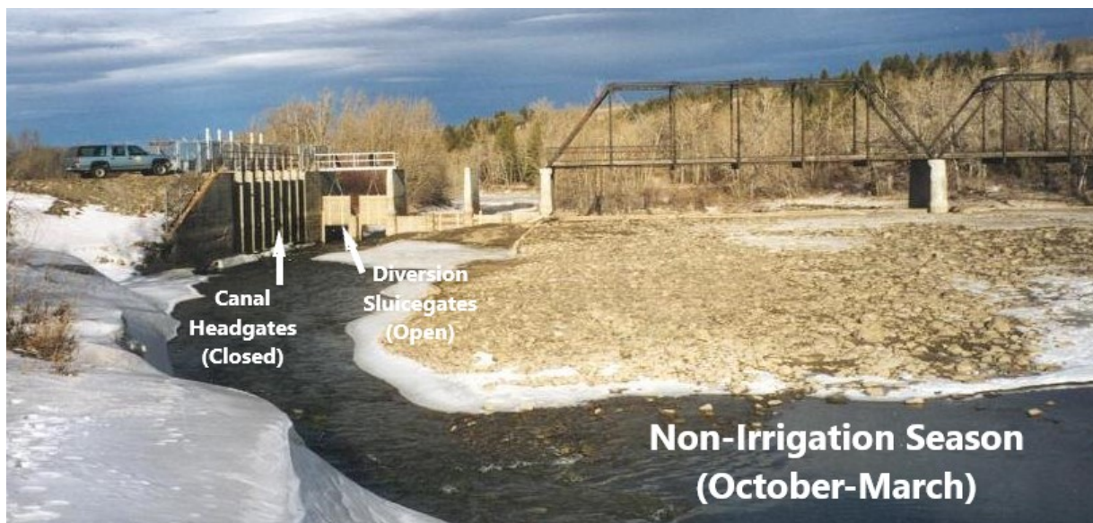
Figure 6. St. Mary Diversion Dam Non-Irrigation Season
