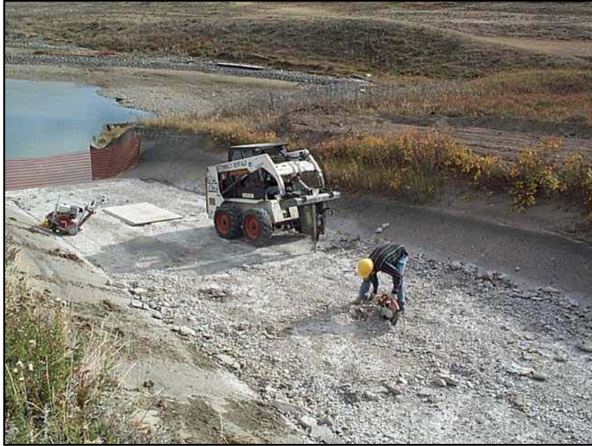
Photo 35. Repairs being made to chute floor of Drop No. 3 during off-season (10/13/04).
