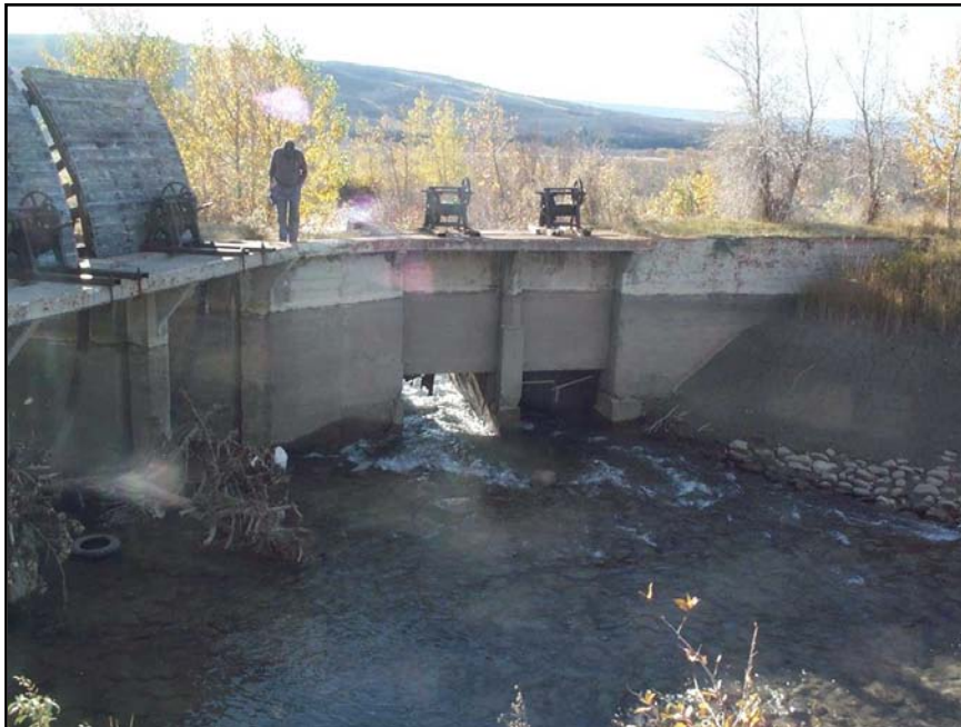
Photo 14. Upstream view of Kennedy Creek wasteway structure during off-season. Note only one gate is open. Check structure is to left. (10/13/04).
