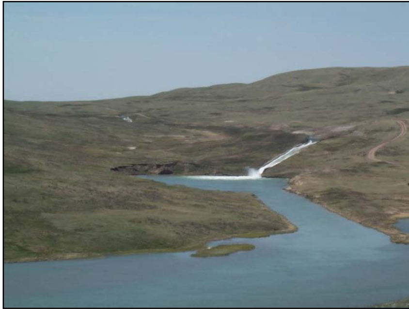
Photo 34. Looking upstream towards Drop No. 2 (05/16/06),
