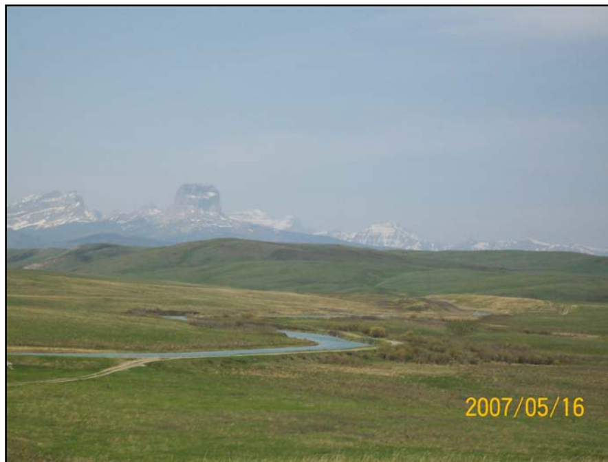
Photo 48. Canal, looking upstream toward Big Cut Slide. Note winding, contour-following nature of the canal alignment. (05/16/07).
