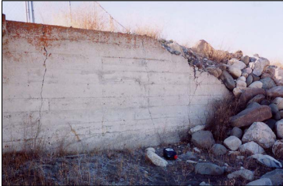
Photo 11. Kennedy Creek side of inlet transition structure (11/11/04).
