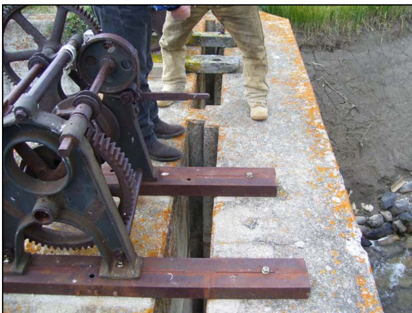
Photo 16. Kennedy Creek wasteway operators (09/25/07).
