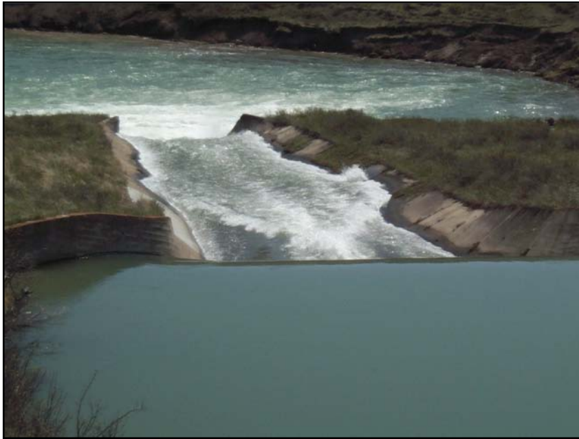
Photo 36. Looking downstream at Drop No. 2 during diversion. Note dramatic change in flow regime. Also see Photo 37 (05/16/06)
