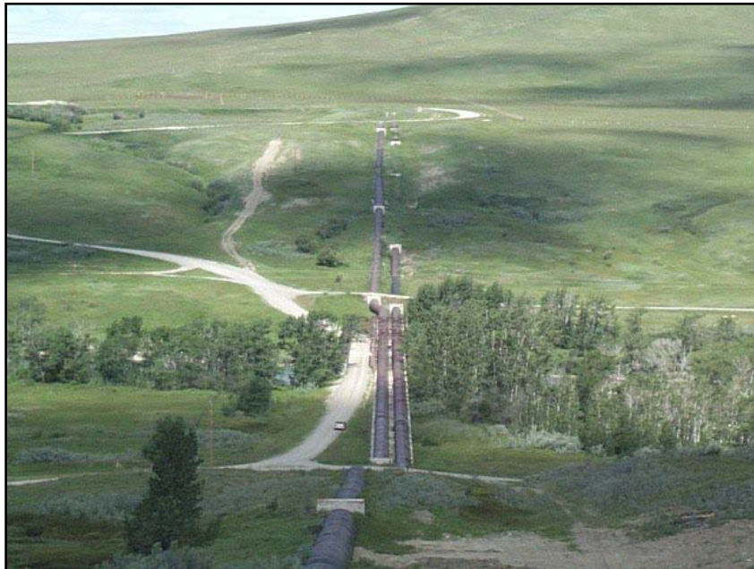
Photo 18. Looking upstream (northeast) along the St. Mary River Siphon crossing (07/04/05).
