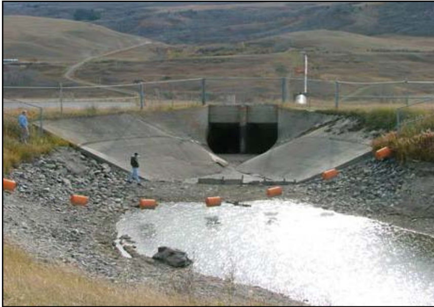
Photo 19. St. Mary River Siphon inlet structure (10/13/04).
