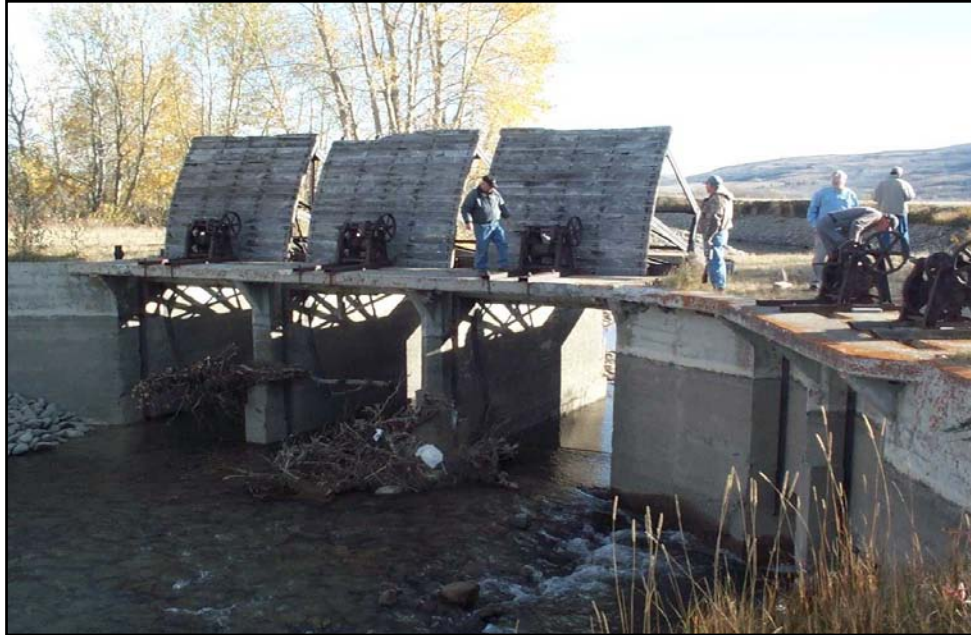
Photo 13. Upstream view of Kennedy Creek check structure during the off-season. Wasteway is located at right side of photo (10/13/04).
