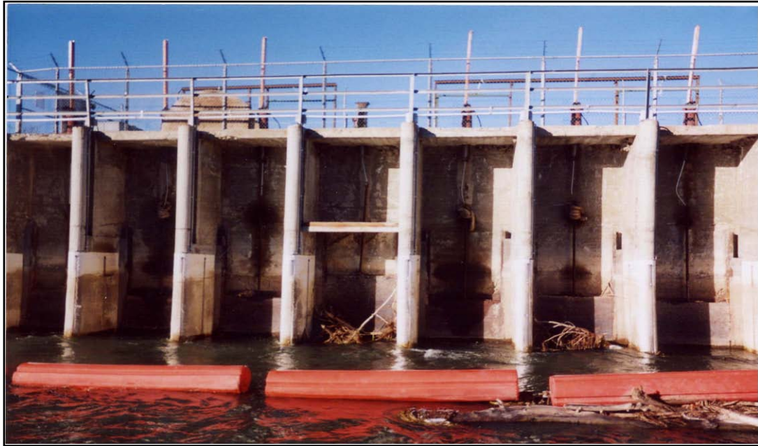
Photo 5. Upstream view of gate openings (11/11/04).
