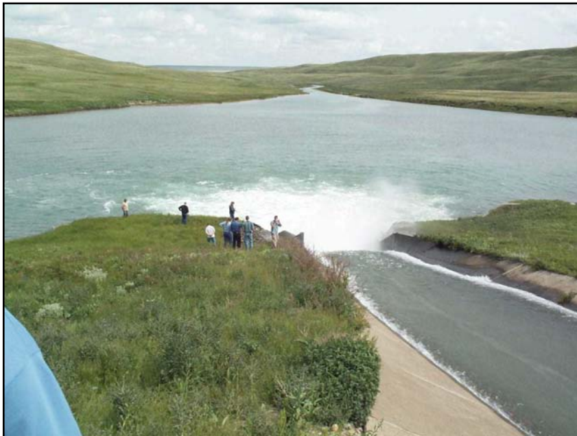
Photo 33. Looking downstream at Drop No. 1 chute and stilling basin (06/24/04),
