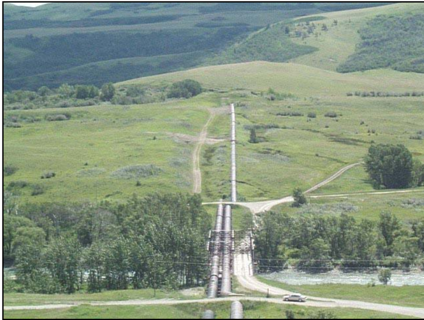
Photo 17. Looking downstream (southeast) along the St. Mary River Siphon crossing (07/04/05).
