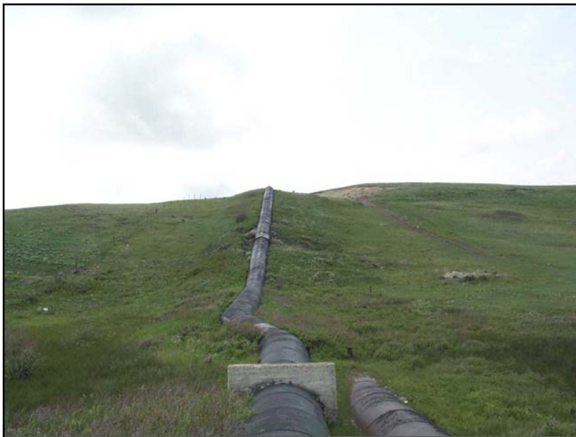
Photo 31. Looking upstream toward inlet of Hall Coulee Siphon (10/13/04).
