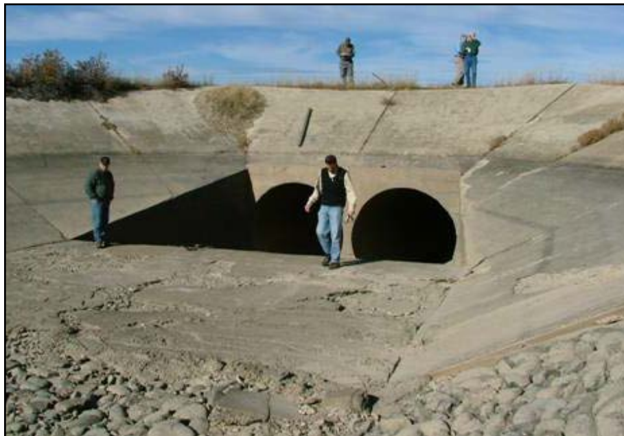
Photo 20. St. Mary River Siphon outlet structure (10/13/04).
