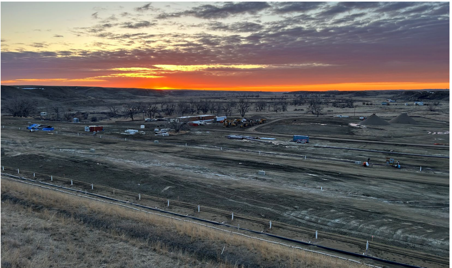
Downstream of Fresno Dam
